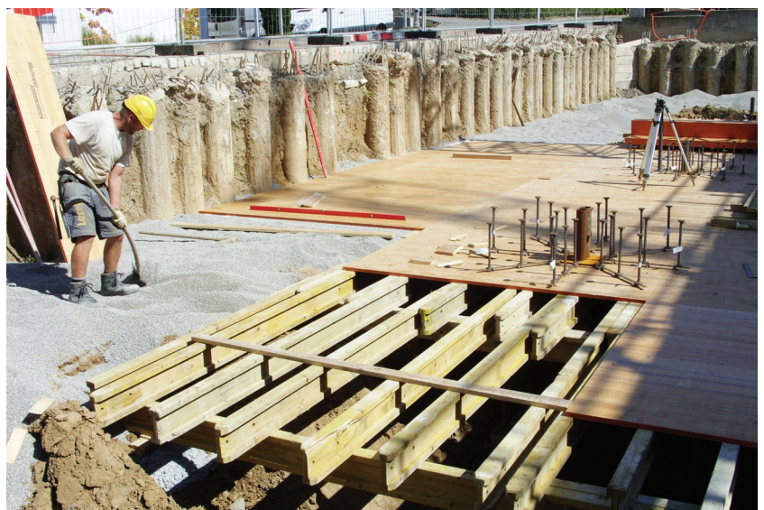
Hofkellerdecke in Deckelbauweise
